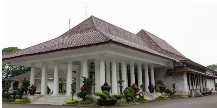
Fig.10. Serang Regent Office Building
