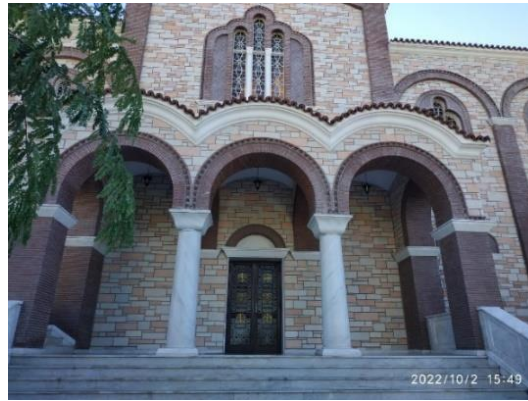
Fig. 20. A Non-linear structure (Church) in a natural environment with few trees and without PnP linear geometries→ No Birds’ nests found Photo by courtesy@Ch. Basdekidou (Article’s author)
